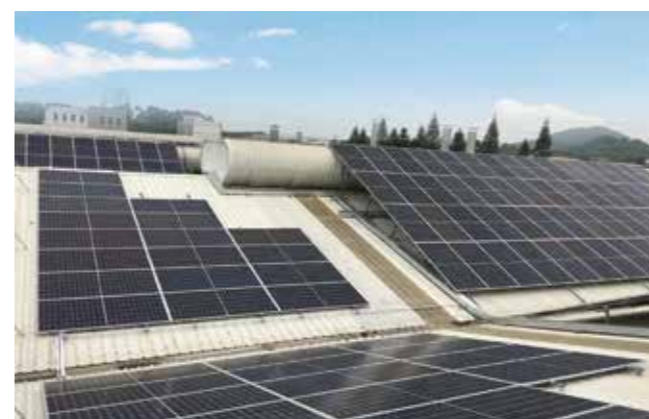
PANYU 1.035MW POWER STATION PROJECT
